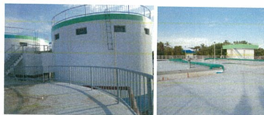
Overview of STP
