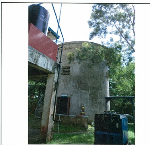
Nabaoy Intake Plant
