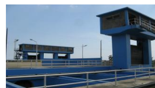
Developed pumping station in the project
