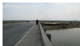
Developed bridge in the project
