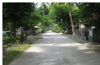
Figure 8: Farm-to-market road constructed
