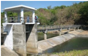
Intake weir constructed in the project
