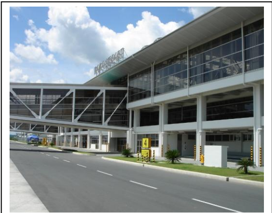
New Iloilo airport (Passenger Terminal)
