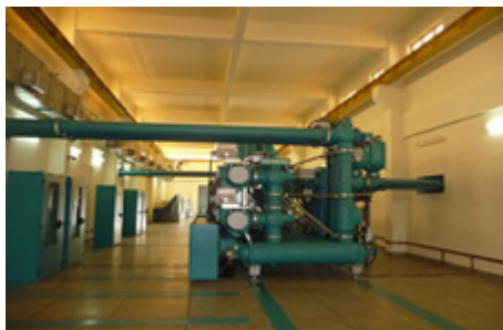
Islamabad University Substation, Bus Bar
