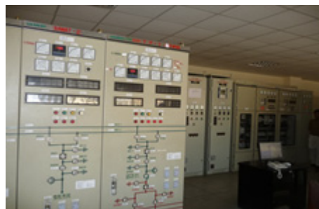
Islamabad University Substation, Control Room
