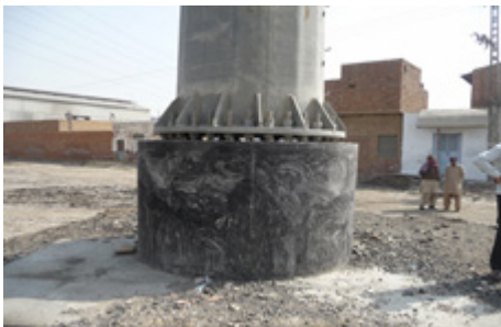
Jamhsoro-Hyderabad T/Line, Foundation work
