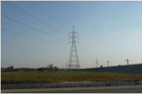
Gatti-Ludewala D/C single conductor T/Line
