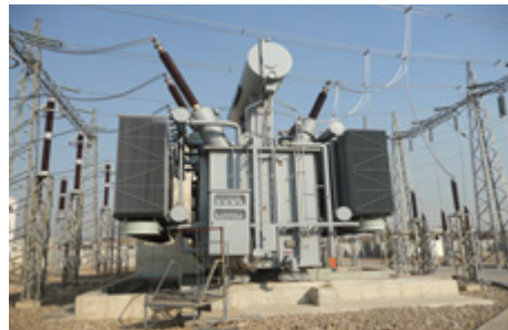
Islamabad University Substation Transformer
