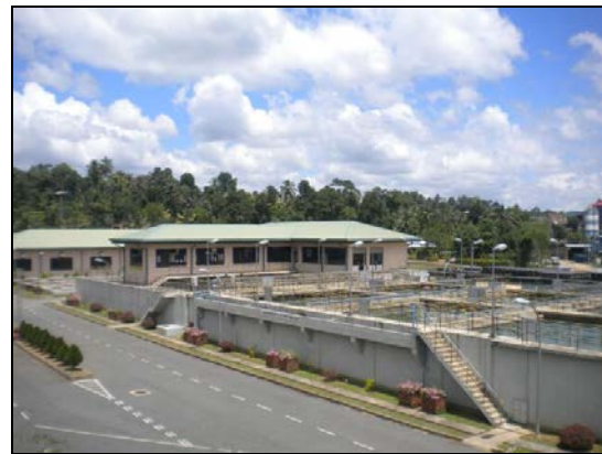
Katugastota Water Treatment Plant
