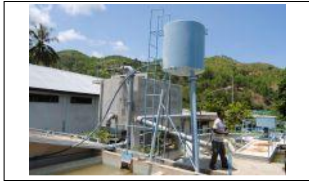
Overall view of Lahane Water Purification Plant
