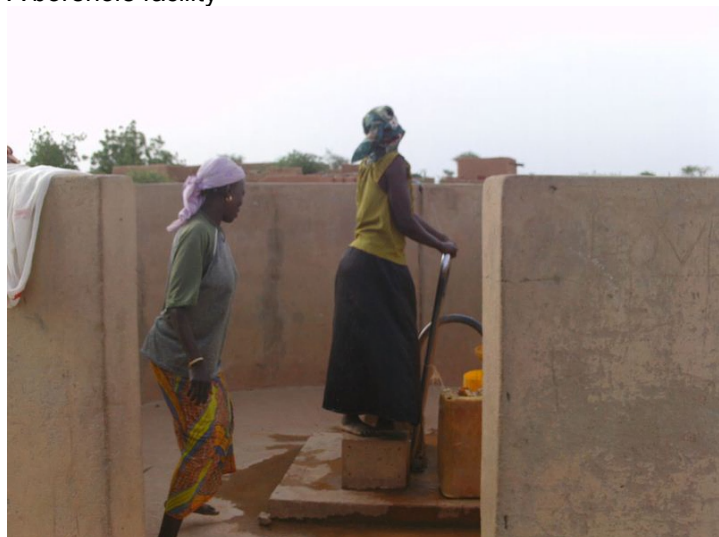
A borehole facility
