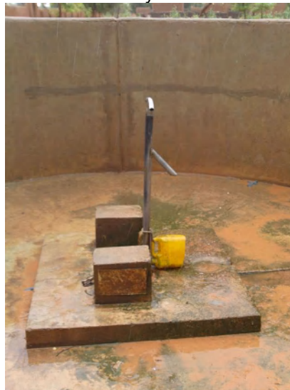
A borehole facility
