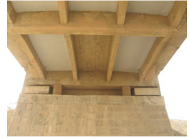
Baring of Emculu Bridge (repaired)
