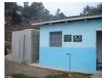
Pump station and water tank (Chimaltenango Department)
