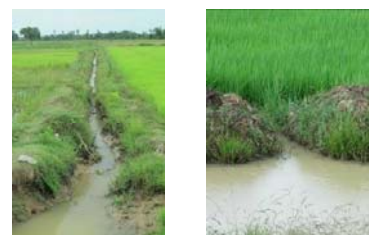
End canals (delivery canals) in the irrigated area (this canals can deliver irrigation water directly into the paddy field.)
