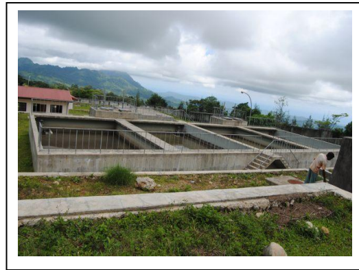
Nugupo Water Purification Plant, Ainaro
