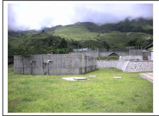
Nugupo Water Purification Plant, Ainaro
