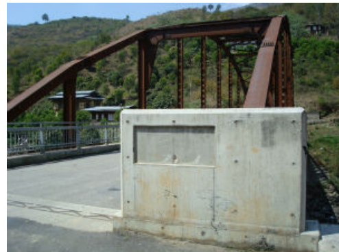
Uninstalled name plate at Tangmachu Br.
