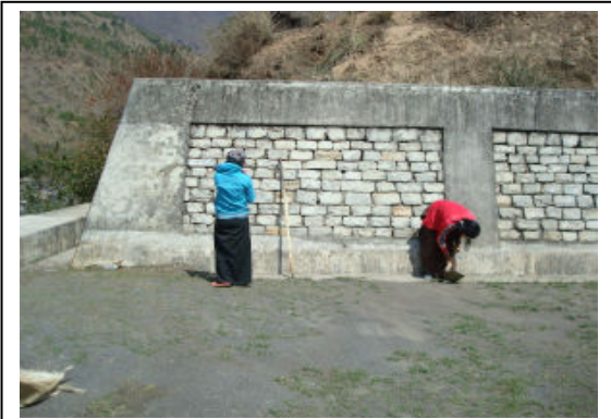
Cleaning bridges by NWF
