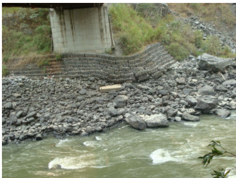
Lowering gabion wall of Wakleytar Br.
