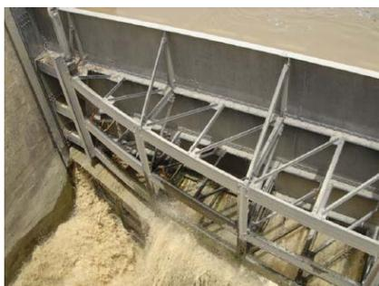
Water leakage from the spillway gate
