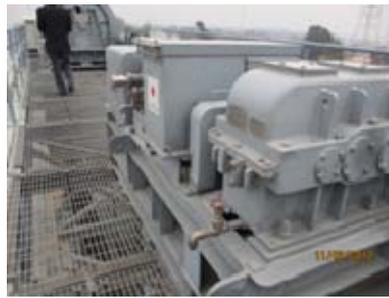
Motorization of gate hoists (operation board set near the apparatus)
