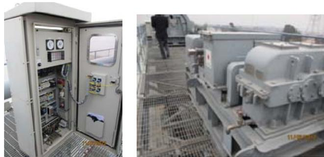
Motorization of gate hoists (operation board set near the apparatus)
