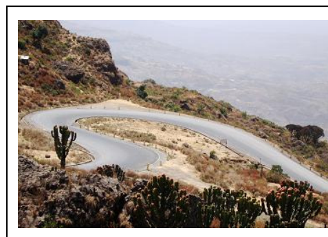
(Abay Gorge and Rehabilitated Road)
