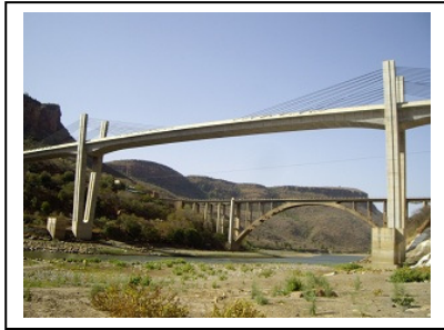
(Abay Bridge (New/front, Old/back))
