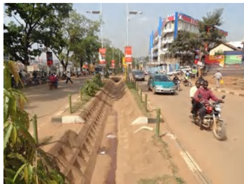
(Well-maintained drainage on Entebbe road)
