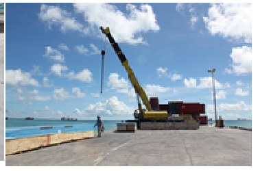
80t Truck Crane Truck in operation
