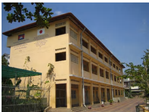
Side view of school building
