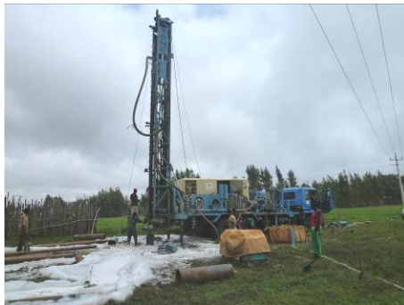
Well Drilling Rig
