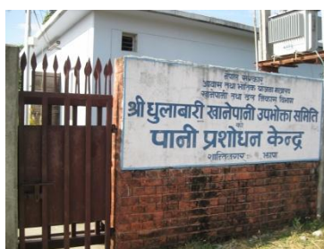
Dhulabari Water Purification Plant (entrance)
