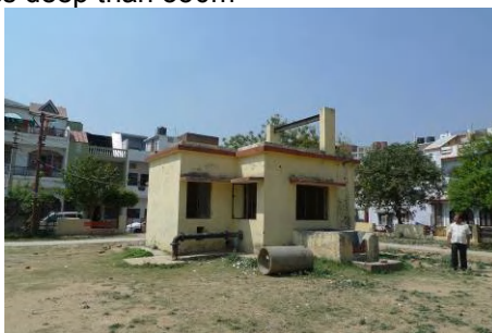
A well constructed by project equipment
