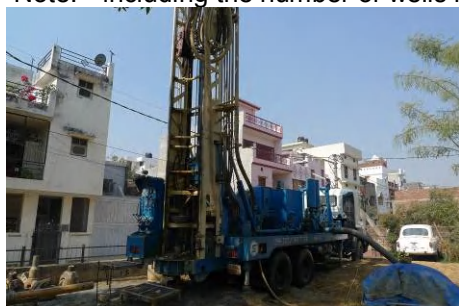
A well being drilled by project equipment
