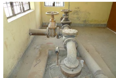
A well constructed by project equipment
