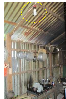
Lighting device installed in a kitchen
