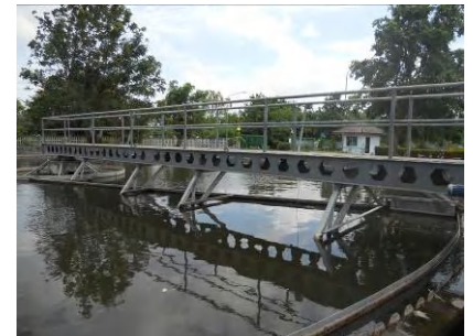
Clarifier Tank at STP
