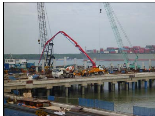
Cai Mep Terminal under construction
