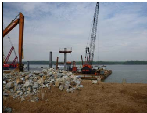
Photo 1: Thi Vai Terminal under construction
