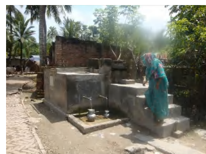
A village women taking water from Arsenic Iron Removal Plant (AIRP) Fulshara Village, Chowgacha Upazila
