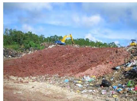
M-Dock Landfill in the cover soil operation
