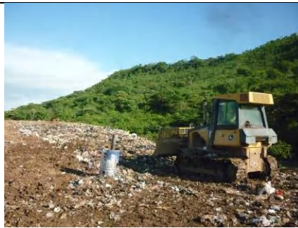
Provided equipment in operation
