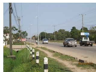
Section that was repaired several times
