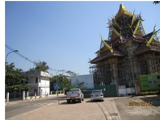
The new shrine being built on Road No. 1
