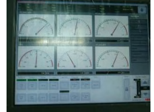
Digital monitor of new exciter system
