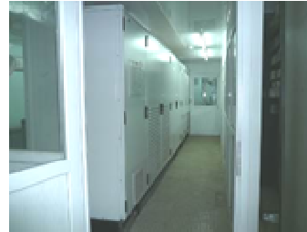
New exciter system procured
