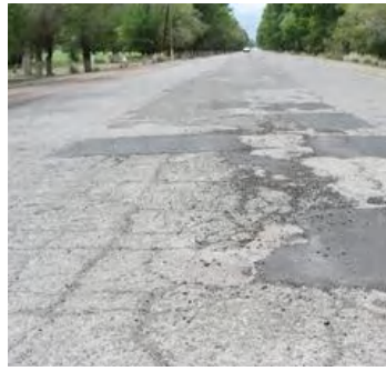
After the repair of BNT road (June 8, 2012)
