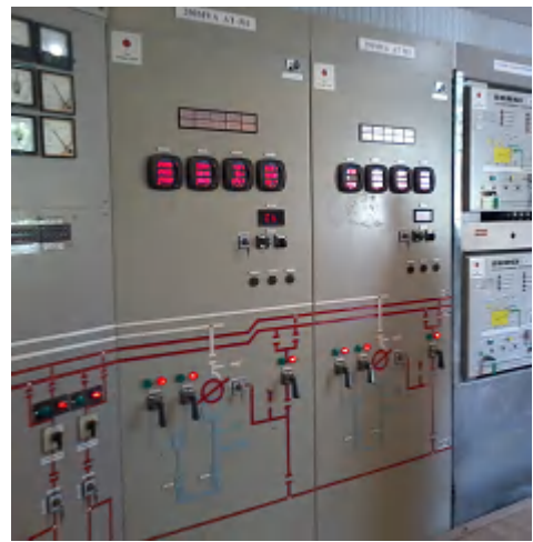
(Control panels for main transforms in the control building)
