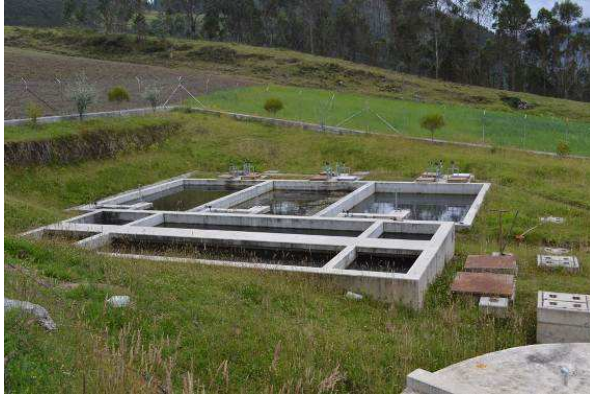
Purifying plant at Zuleta
