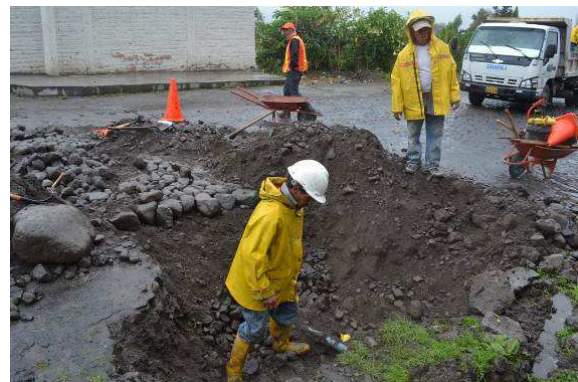
Works for water leakage prevention
