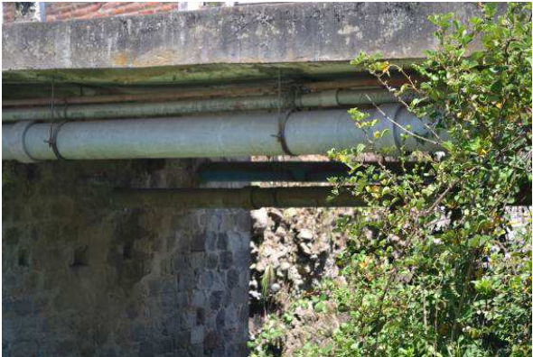
Conveyance pipe at Esperanza
