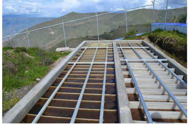
Rapid Filtration installed at Aloburo Purifying plant
