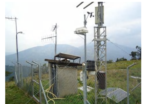
Monitoring Point in the Mountain
