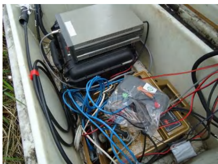
Seismograph installed at the Monitoring Point
