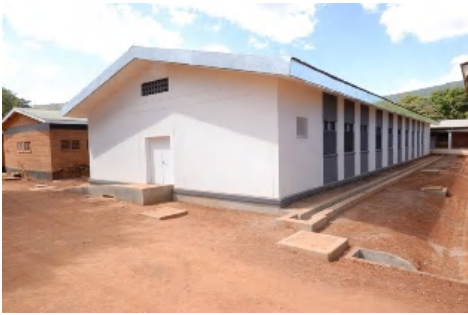
Maternity Ward in Rumph District Hospital
