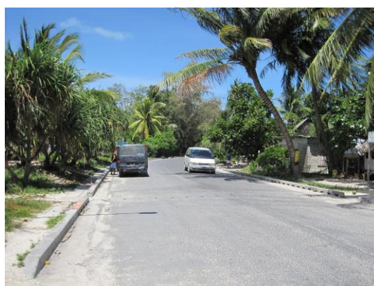
Road Section Improved in the Project
