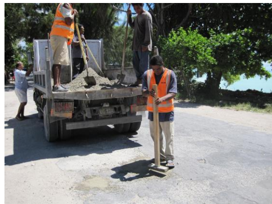
Photo 3: Road Maintenance Work (Non-Project Section)
