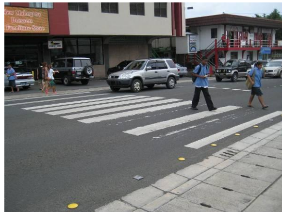
The Arterial Road after its rehabilitation (Section A: Downtown Koror)
