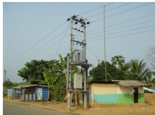
Upper Denkyira District Facility Installation
