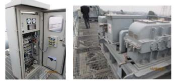
Motorization of gate hoists (operation board set near the apparatus)
