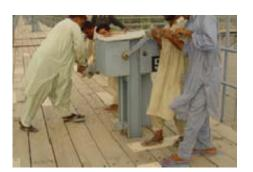
Water leakage from the spillway gateManual operation for the gate(It is impossible or difficult for some gates to be opened or closed due to damage to the gate hoists.)
