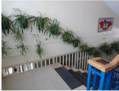
(Exchanged flooring to strong material)
