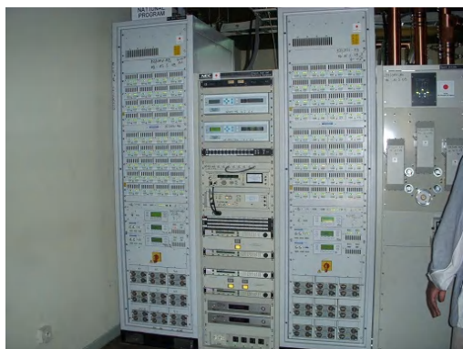
Transmission Equipment for Ngaoundéré Station
