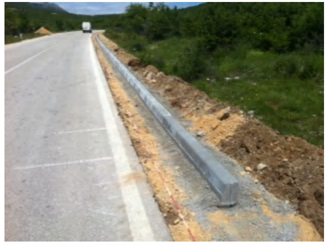
Reinforcement work of shoulder
