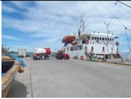
A jetty: Cargo handling by a trailer has become easy because of the sufficient width.
