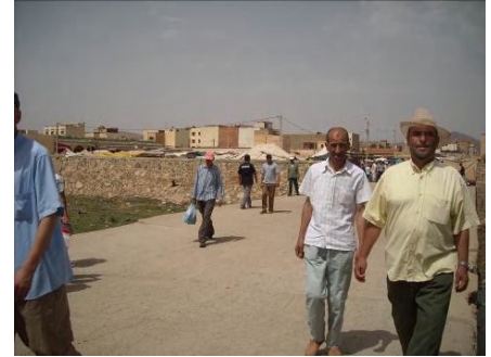
Arterial road constructed by a project for construction of river canal (Murilt)
