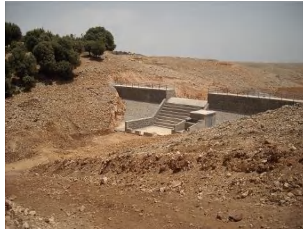
Masonry Dam (Aharal Dam)
