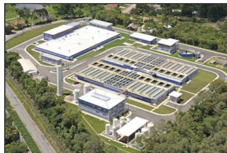
Miringuava Water Treatment Plant
