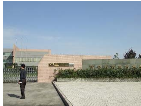
Xi'an No.3 Wastewater Treatment Plant
