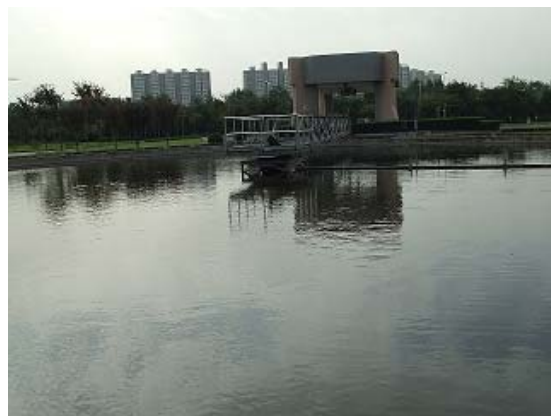
No. 3 Wastewater Treatment Plant
