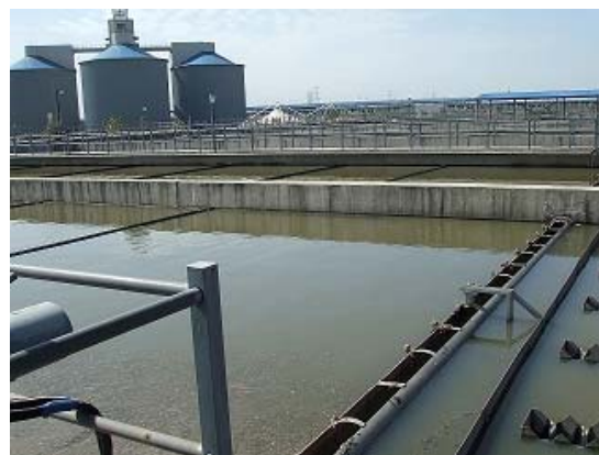
No.4 Wastewater Treatment Plant
