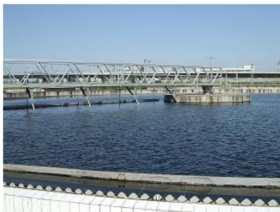
No.4 Wastewater Treatment Plant
