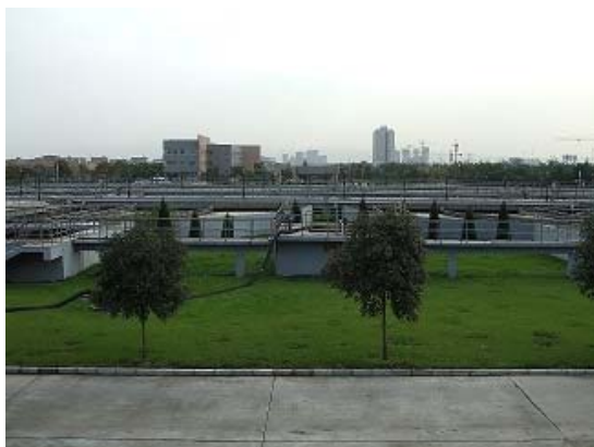
No. 3 Wastewater Treatment Plant
