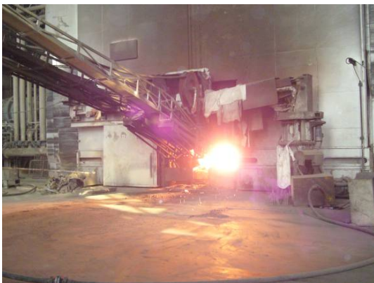
Electric Arc Furnace (EAF)
