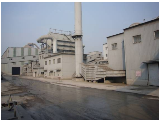
Steel dregs treatment plant
