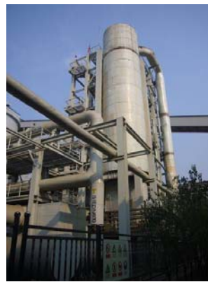
Desulphurization and HCN Removal Plant
