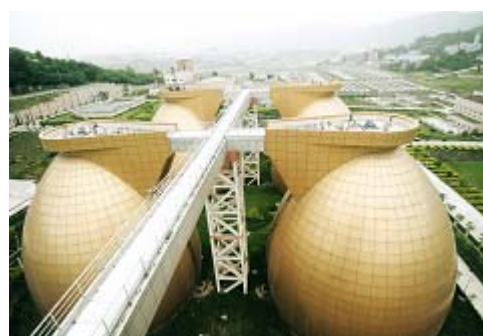
Jiguanshi Wastewater Treatment Plant Digestion Tank
