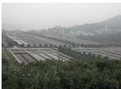
Overview of sedimentation pond and biological reaction pond
