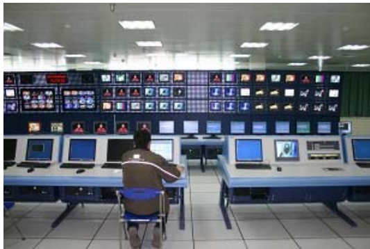
Jinan TV Station: monitoring room
