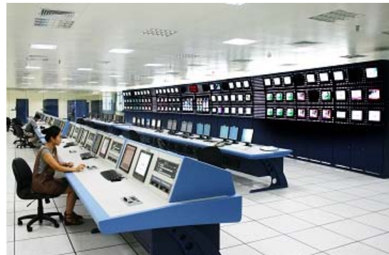
Jinan TV Station: monitoring room
