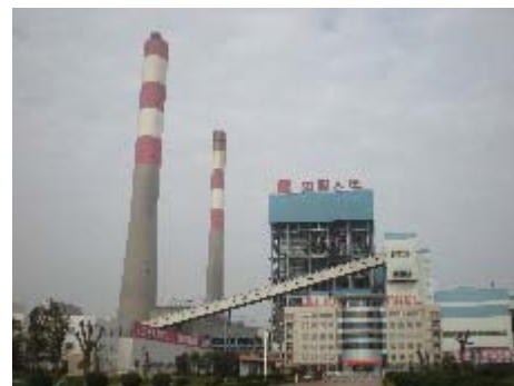
Hancheng No.2 Thermal Power Plant
