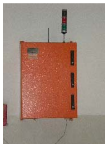
Network Equipment for Online monitoring system
