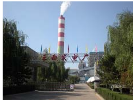
Wangqu Thermal Power Plant
